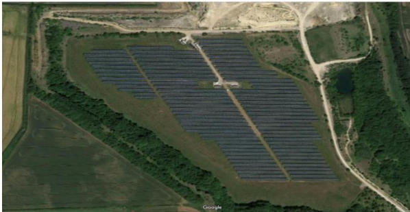
Figure 1.1 — Solar PV Farm in Bolsover
